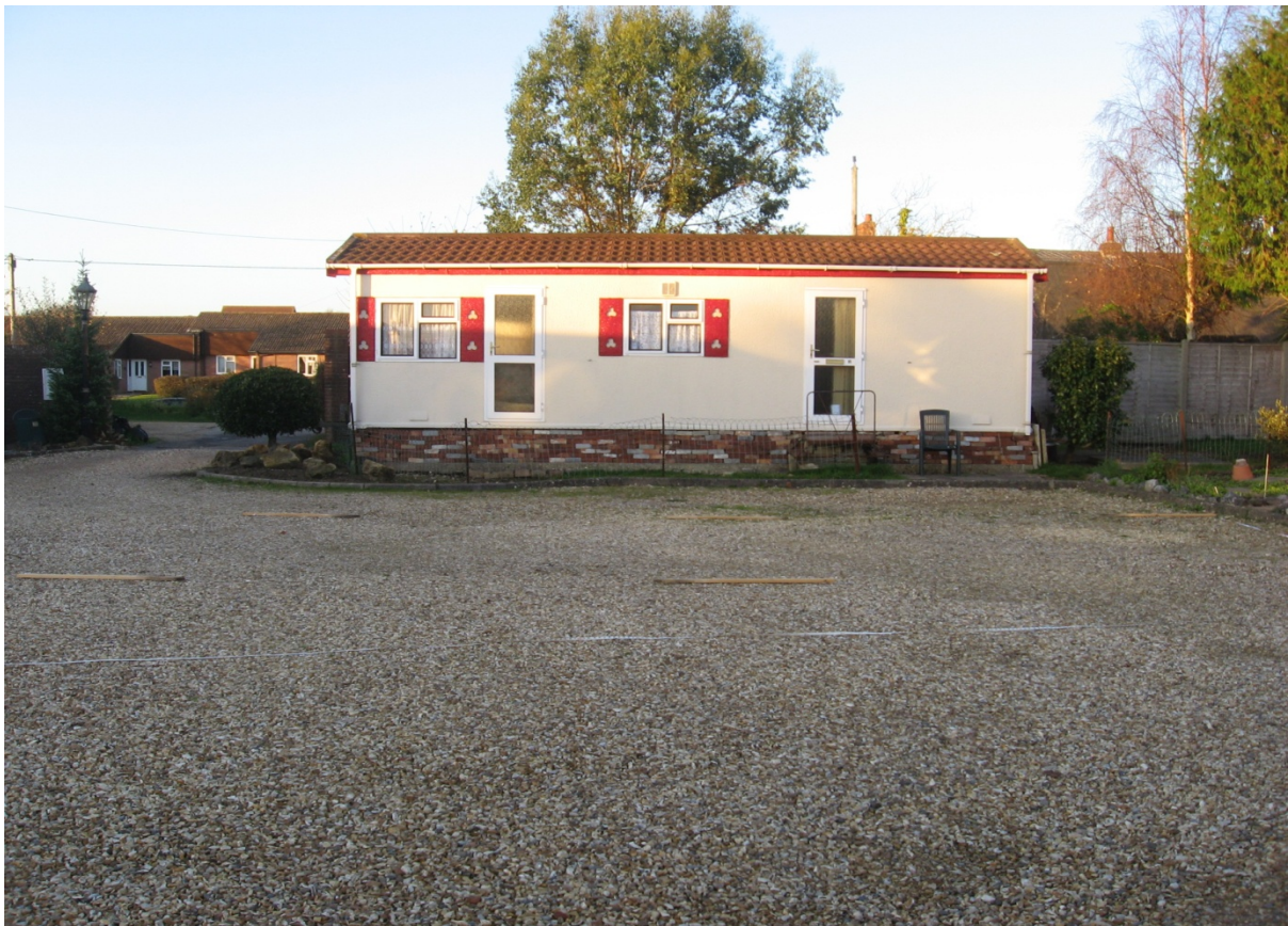
2. Showing home 14 with area of proposed development in the foreground.
